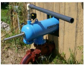
cleaning itself, filtered water continues to flow. This also eliminates the need for standby filters and elaborate valve schematics, frequently needed with other types of filters.
